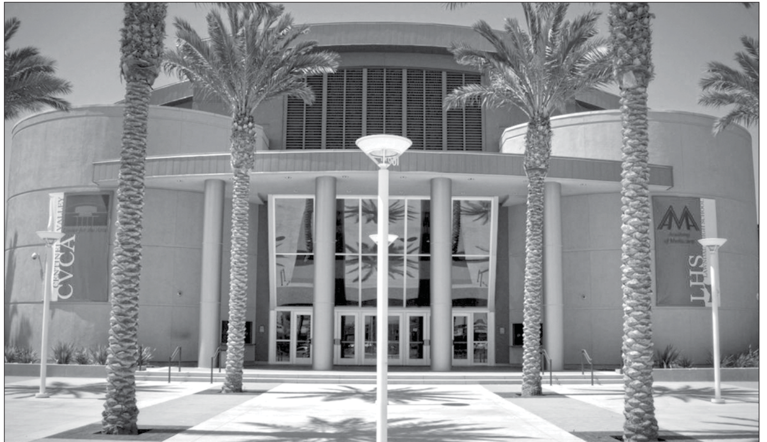
The new Centinela Valley Center for the Arts, provides educational facilities for theater students of Lawndale High School's Academy of Media Arts. Photo by www.christopherbarnesphotography.com
